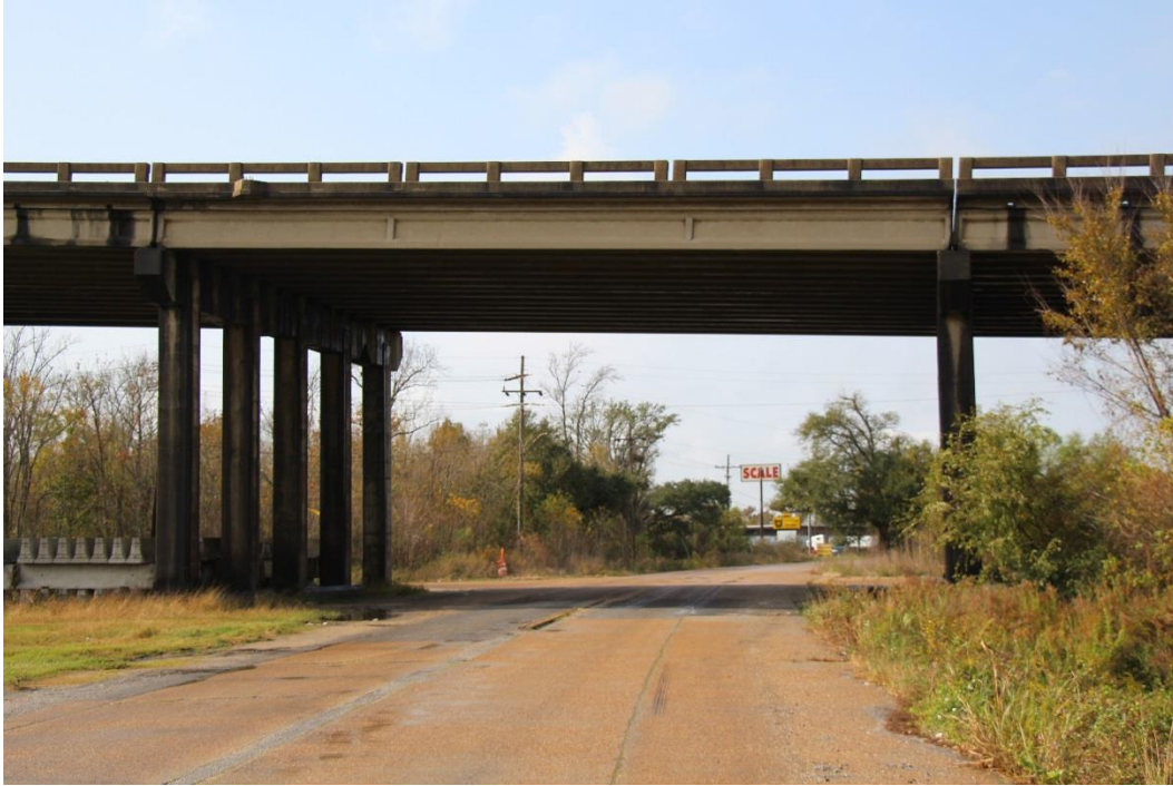
Historic Fabric Photo 3: Typical prestressed concrete girder approach span.
