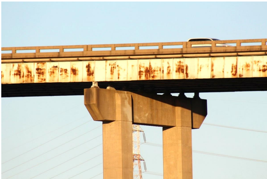
Historic Fabric Photo 2: Typical steel girder approach span.
