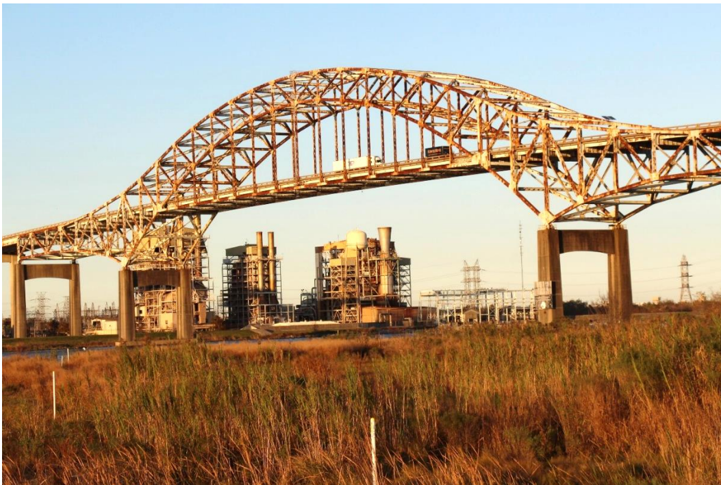
Character-defining Feature Photo 2: Design and construction of a cantilever steel Warren truss with tied-arch suspended span. The Warren truss features diagonal members to withstand both tensile and compressive forces, and added verticals for bracing.
