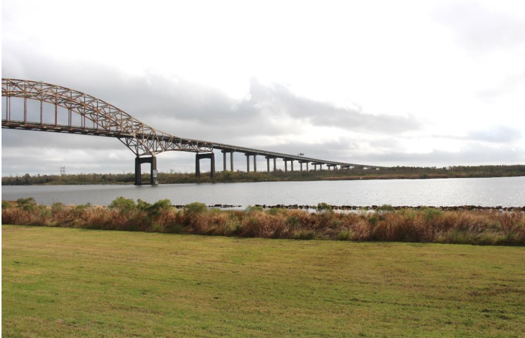
Condition Photo 13: Condition of waterway banks, each side of waterway; both sides of the waterway are protected with levees.
