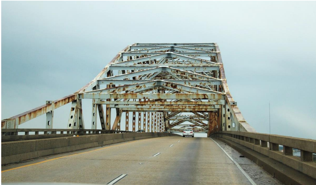
Historic Fabric Photo 1: Concrete deck and original concrete railings.
