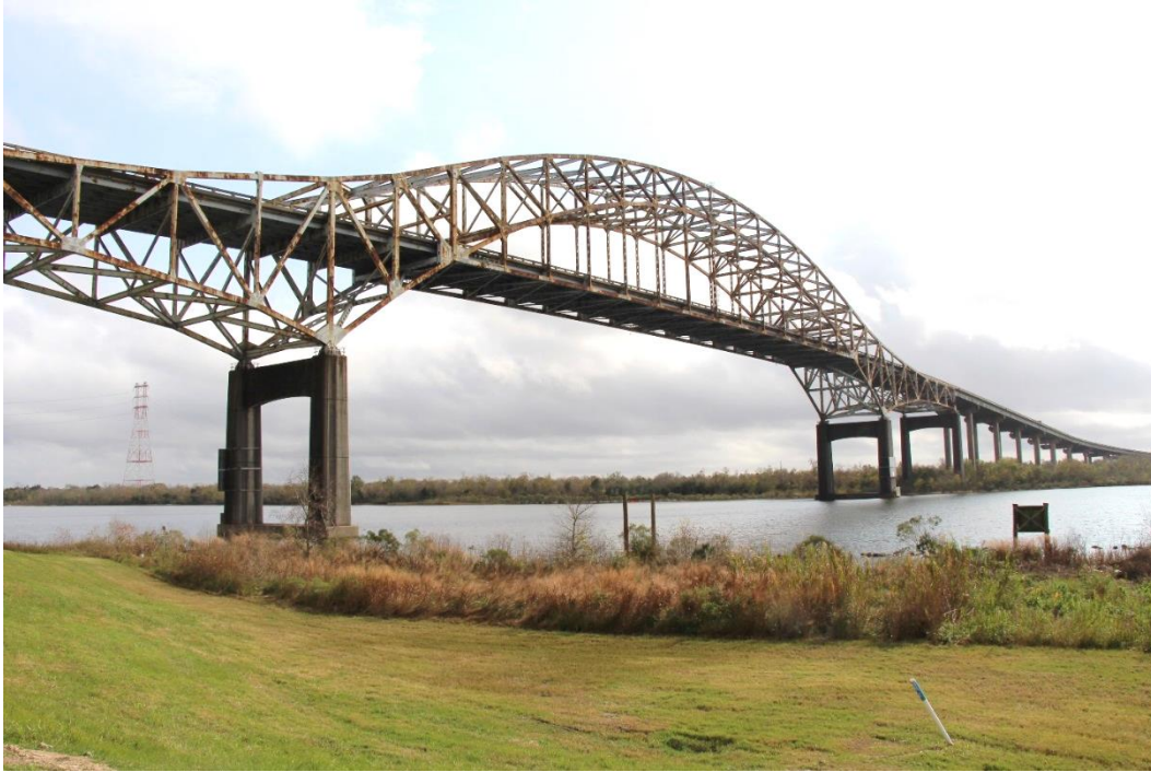
Character-defining Feature Photo 1: Design and construction of a cantilever steel Warren truss with tied-arch suspended span. The Warren truss features diagonal members to withstand both tensile and compressive forces, and added verticals for bracing.
